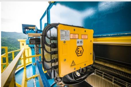
Explosion-proof switch boxes are designed by the crane technology experts in Künzelsau and manufactured for crane systems worldwide.
