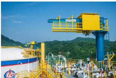
Even if it does not look like it on this photo: LNG hoists are often exposed to wind and weather for years before they are used again. The enclosure protects the wire rope hoists.
